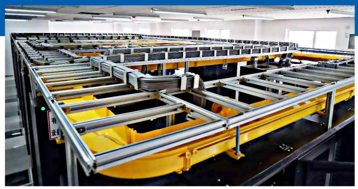
Cable runway is vital part of cable management of horizontal and backbone cable in IT infrastructure. Lepin offers runway and accessories, which are made of
