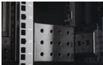
U height indicator vertical rail.
